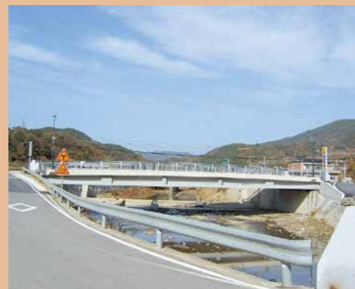
CHA HANG BRIDGE (大韓民国・SPC合成桁橋)
